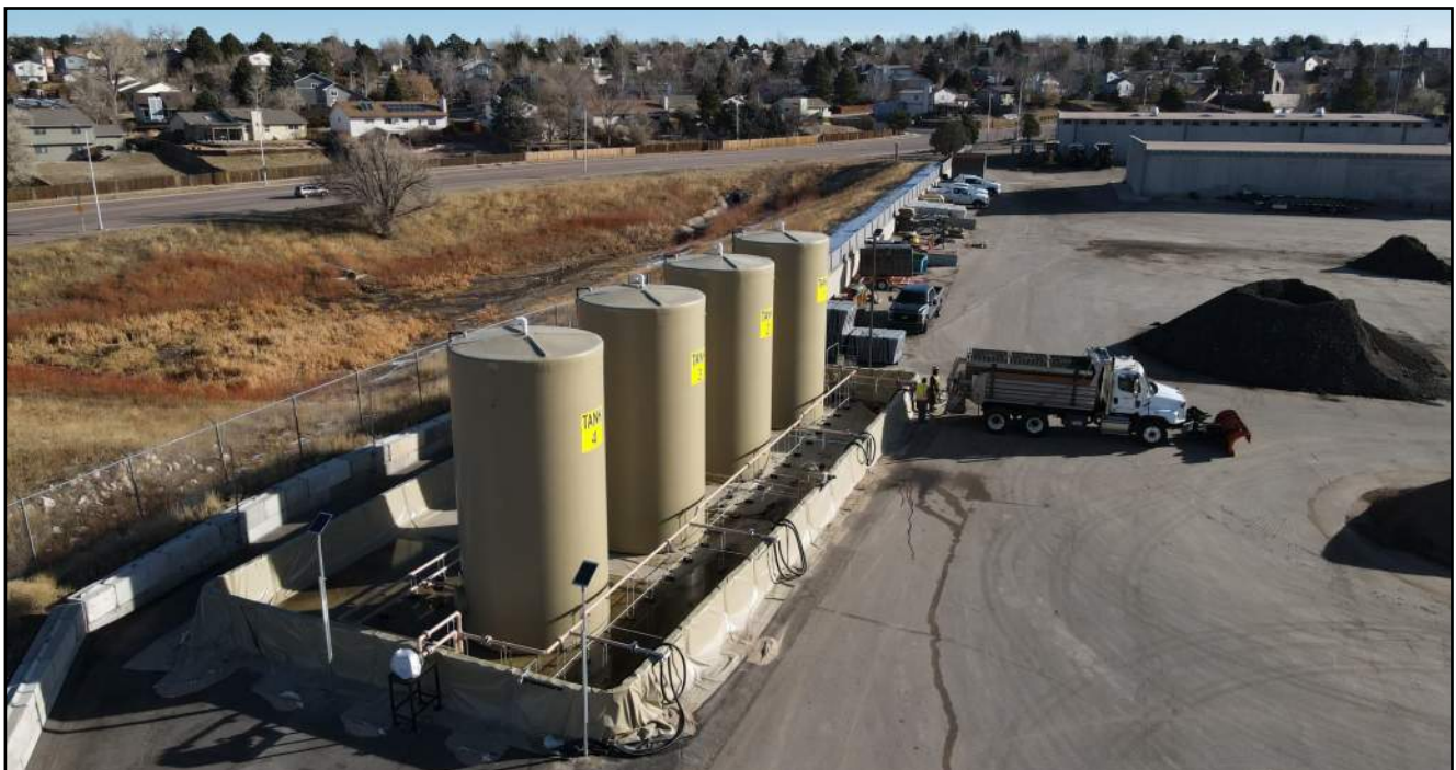
Above: New storage for de-icing materials at the Briargate facility for use by the in-house crews during snow operations.
