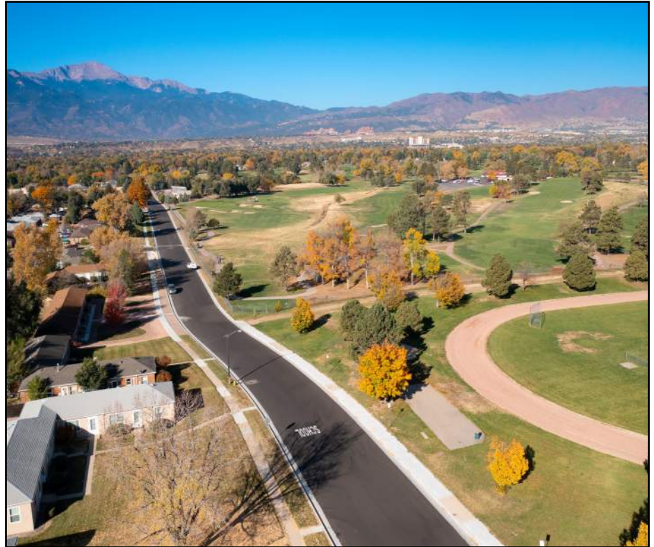
Above E Caramillo Street was repaved with the 2C program during 2023.
