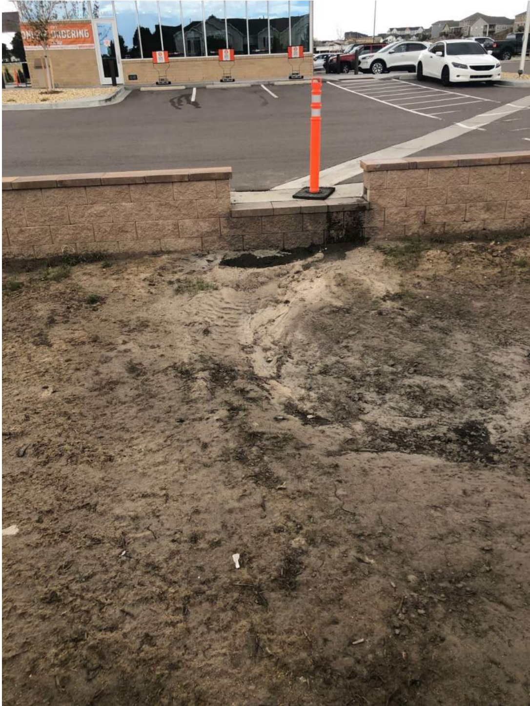
Field identified inlet location into west forebay
