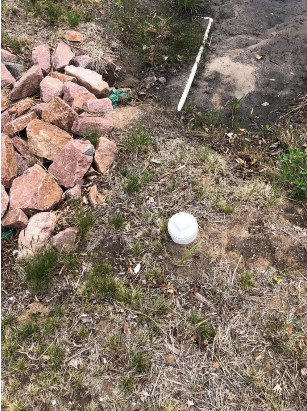
Underdrain connection to outlet structure
