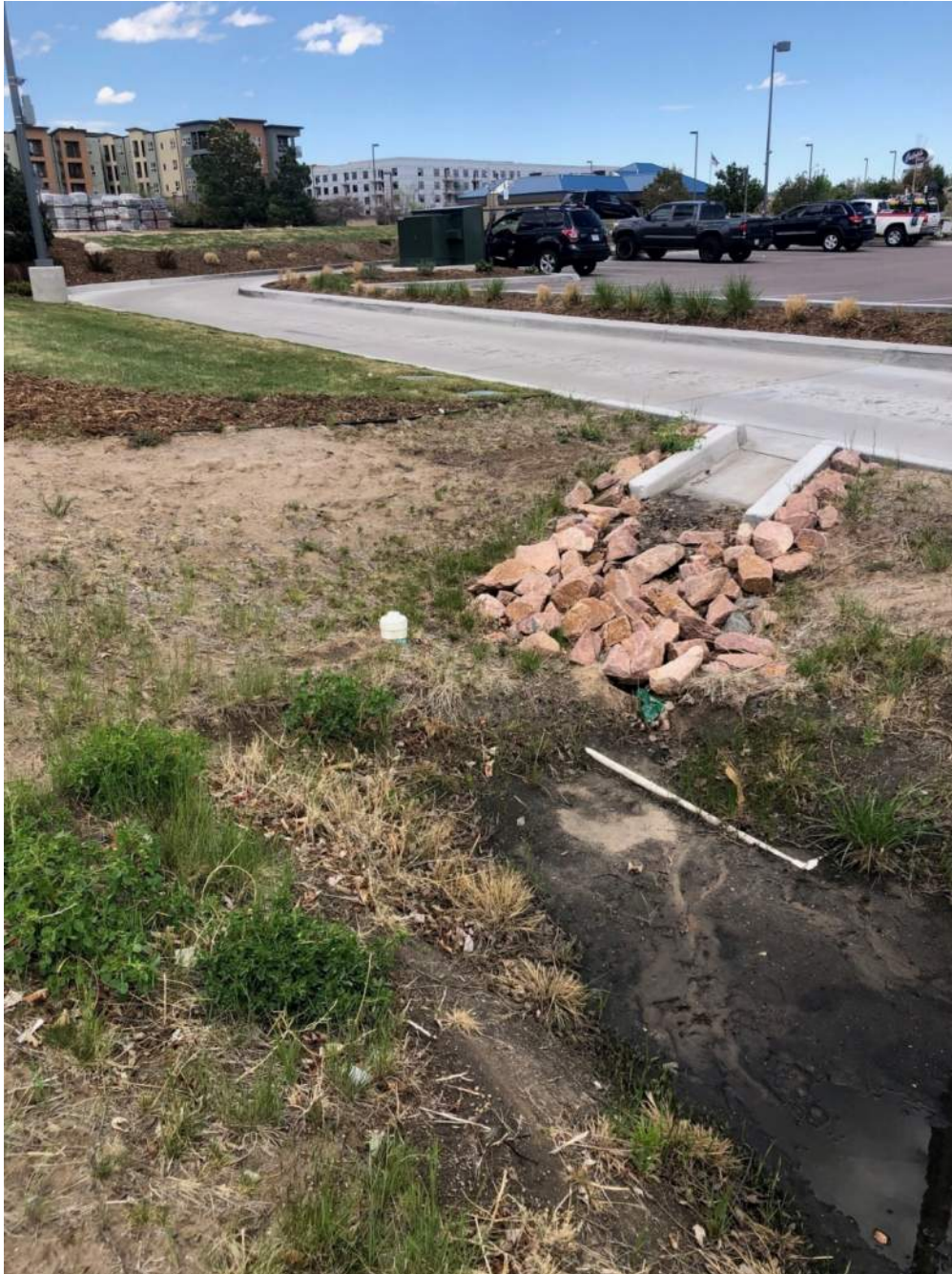
Emergency Overflow / Infiltration Media Example 2
