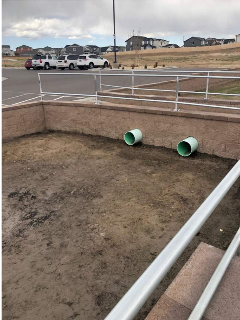
Drainage pipe under walkway connecting forebays
